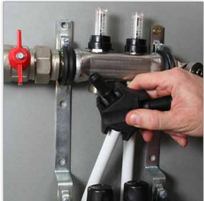
MLC pipework bevelling
